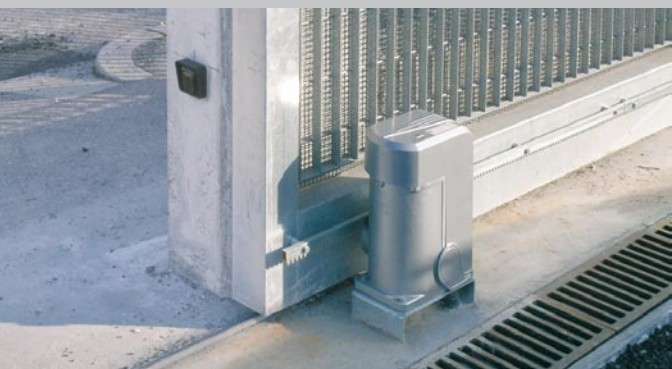
Installation of the operator
